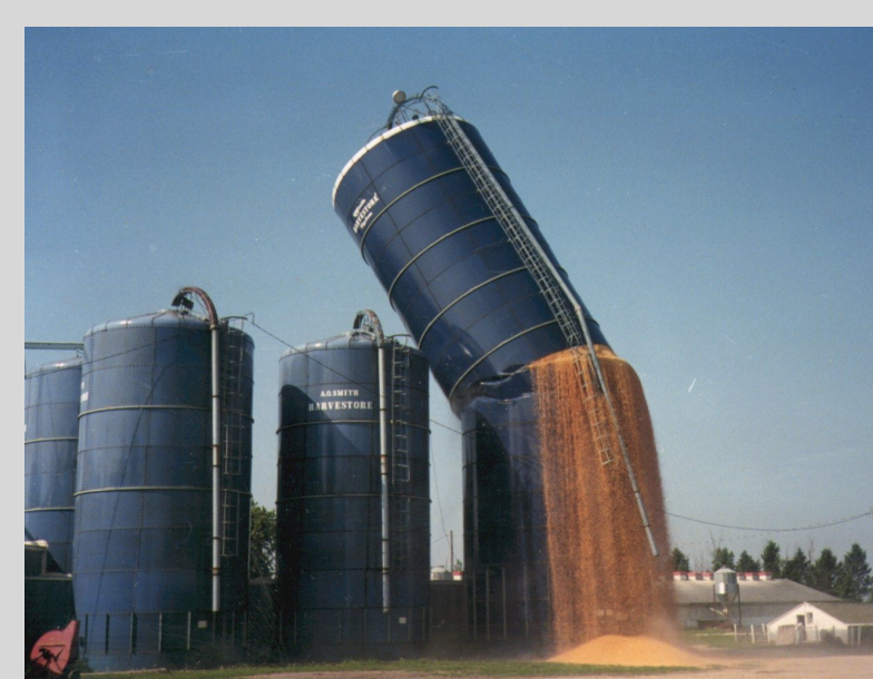
Figure 2: A collapsed silo containing granular material.
